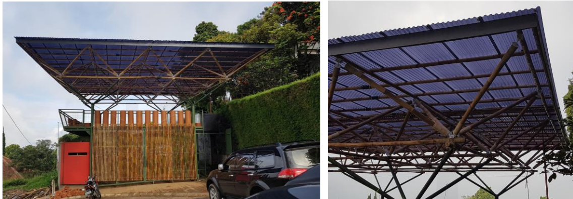
Fig. 8. Implementation of Bamboo Space Frame
